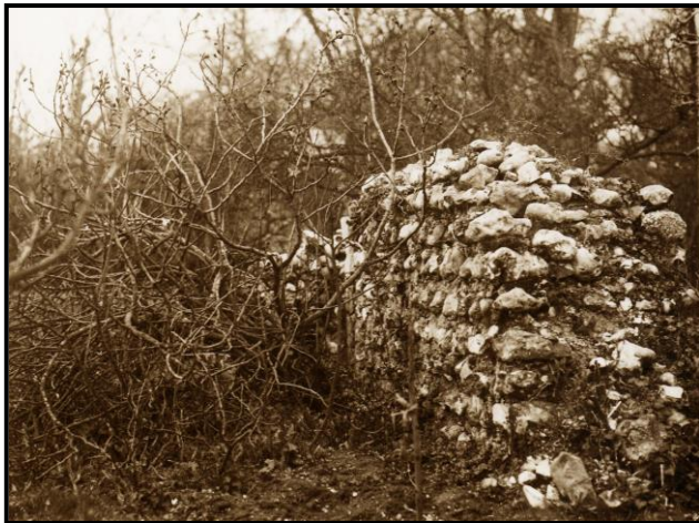
A section of one of the walls of the church in 1940
